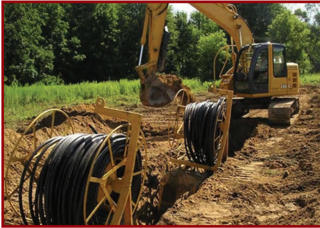
Horizontal geothermal field has nearly 46 miles of HDPE pipe. Pond loop installation: pipes are floated into place then filled with fluid.
