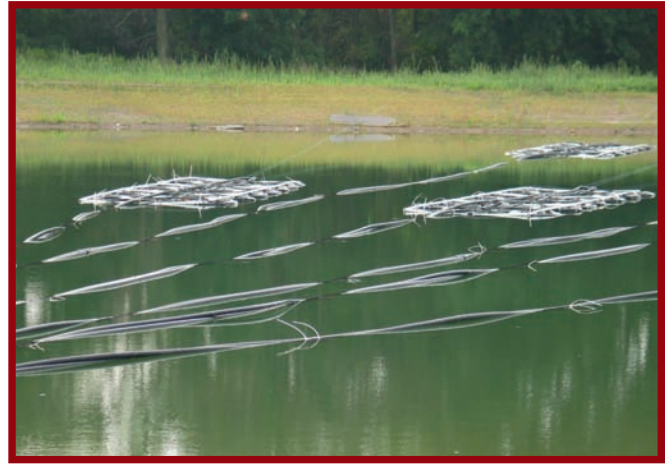
Horizontal geothermal field has nearly 46 miles of HDPE pipe. Pond loop installation: pipes are floated into place then filled with fluid.
