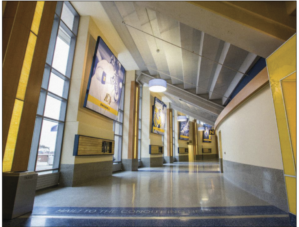
Large graphics on the outside walls are illuminated with metal halide spotlights from across the corridor, and are accentuated by a luminous vertical glowing LED element. LED recessed downlights highlight the curvature of the arena and the new and renovated spaces.
