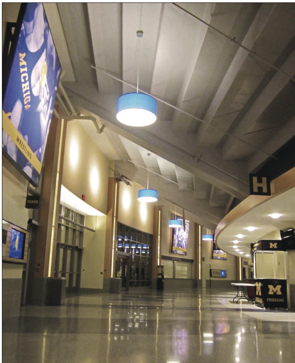
These custom "drums" have compact fluorescent lamps.
