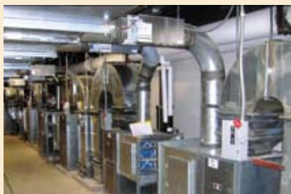
This view of the mechanical room shows the geothermal water source heat pump piping system.
