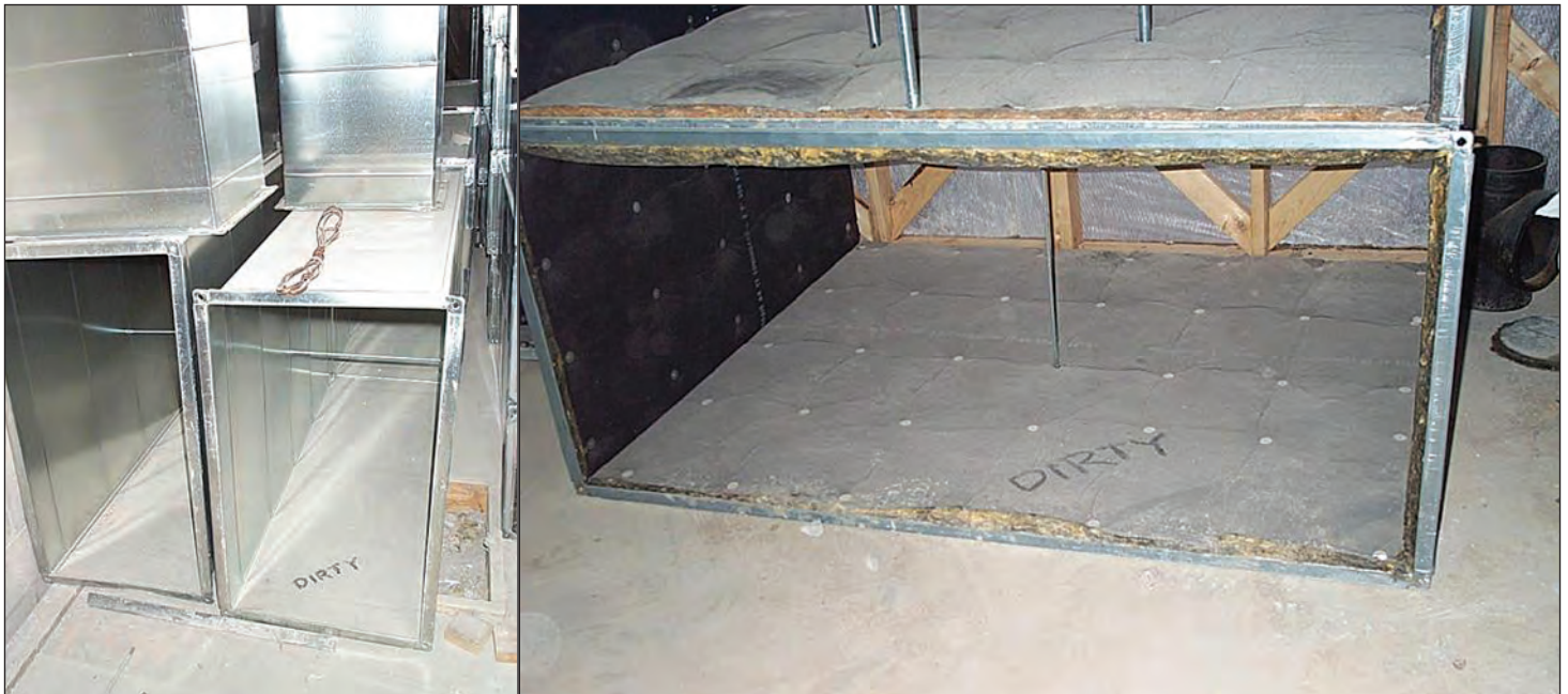
As shown above, improperly staged ductwork allows dirt to accumulate on the duct interior. By helping to prevent this and similar conditions, building commissioning boosts indoor air quality and improves the overall health of a building.
