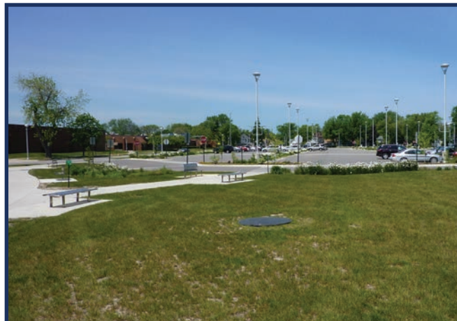
The parking lot is sloped to direct water to green islands, where vegetative filters and groundwater infiltration treats the runoff.
