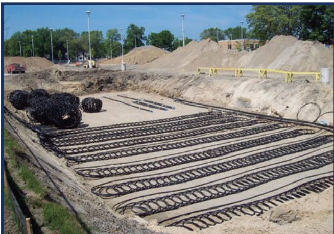
Two hundred and seventy slinky coils were buried 8 ft (2 m) below the 97,590 ft 2 (9066 m 2 ) parking lot.
