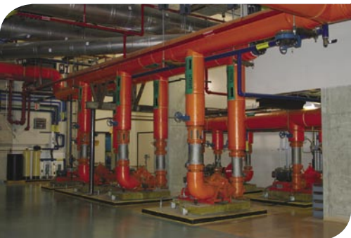
Washtenaw Community College Central Energy Plant
